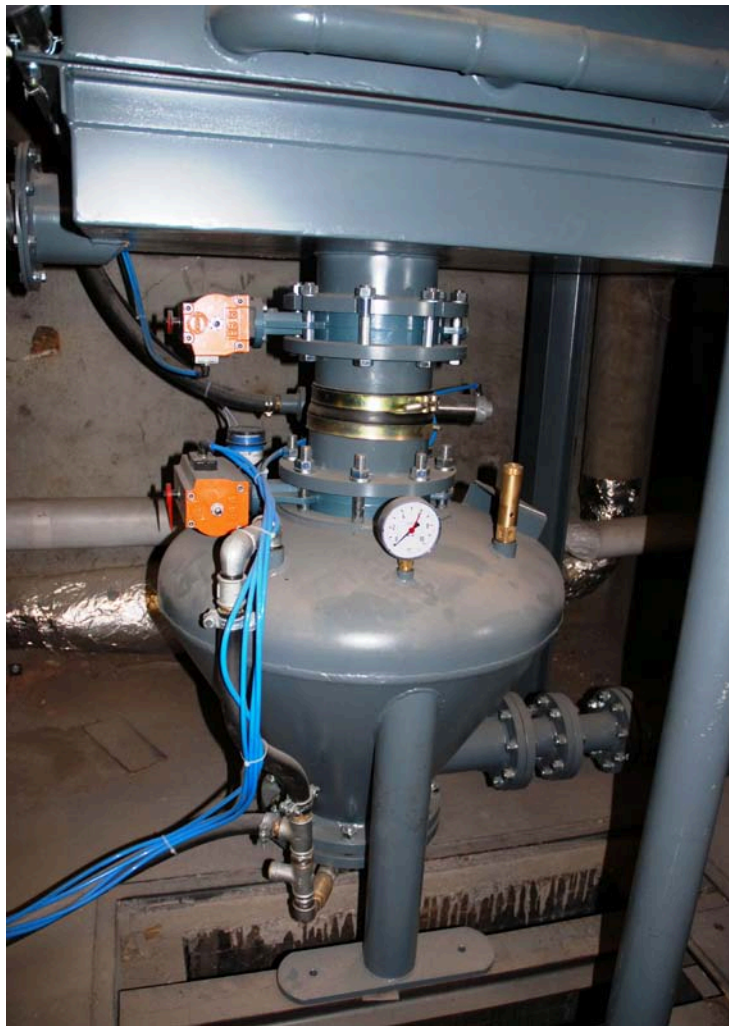
Fig. 9 Oscillating Cooling Conveyor (7 on top) with Sender
