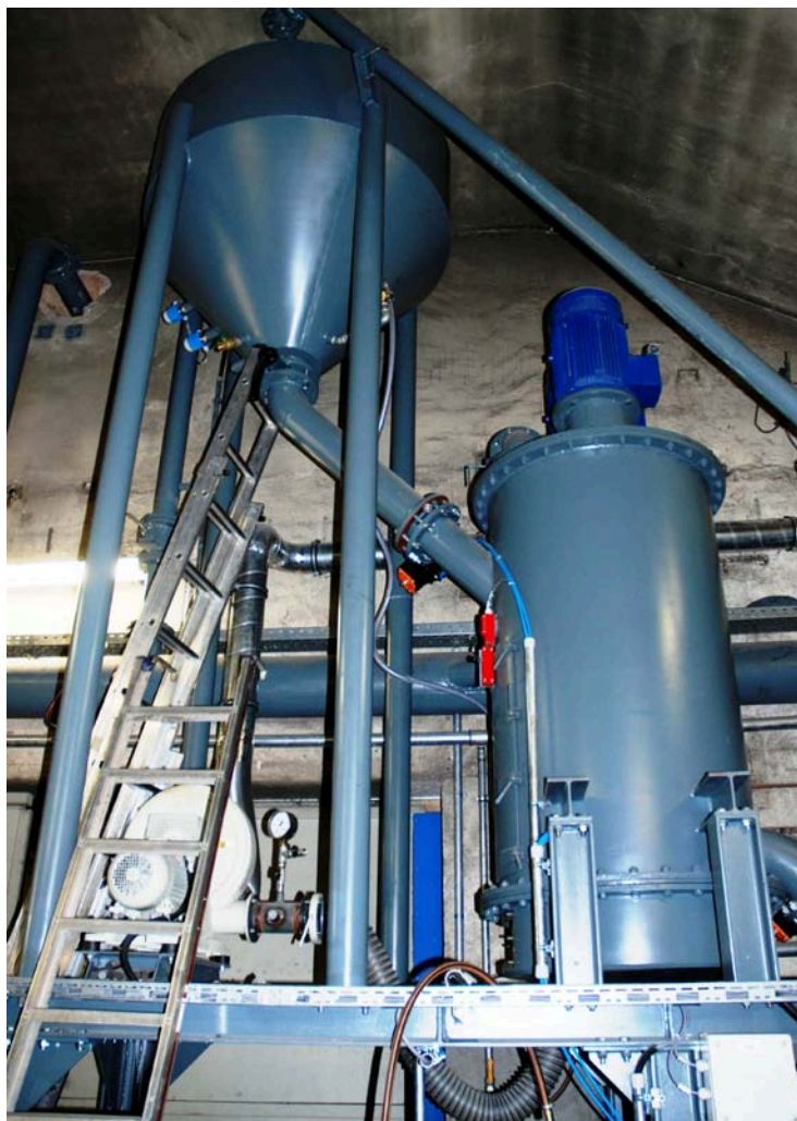
Fig. 4 Surge device (5 top left) and cleaning unit (6)
